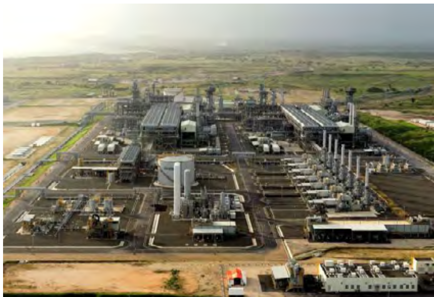
Exxon Mobil PNG's LNG plant near Port Moresby Foto: (C)2014 (Richard Dellman/AdvantagePNG); RNZ 5.12.2018
